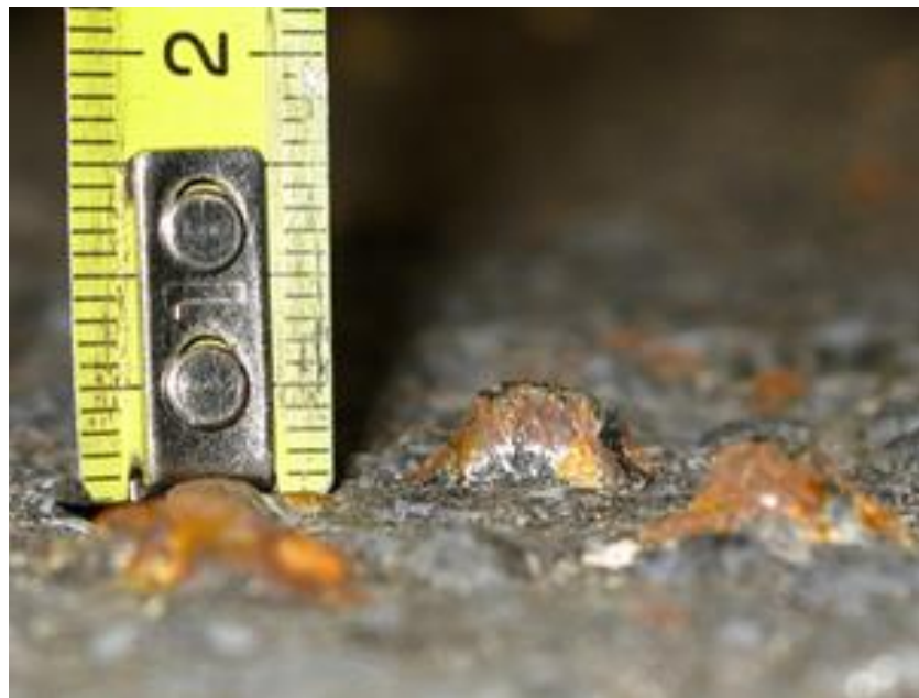
Figure 10. Steel slag aggregates protrusion after long pavement wear by studded tyres (Viman & Gustafsson, 2015)
