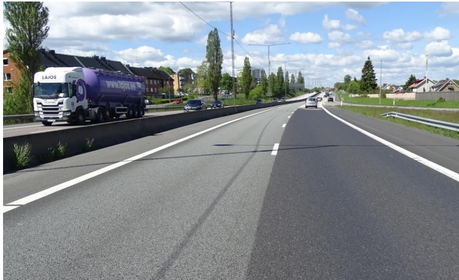
Figure 13. Double-layer PA with steel slag aggregate in the top layer on E4 in Huskvarna, Sweden (right lane only). Exposed to high volume of heavy trucks; four years old
