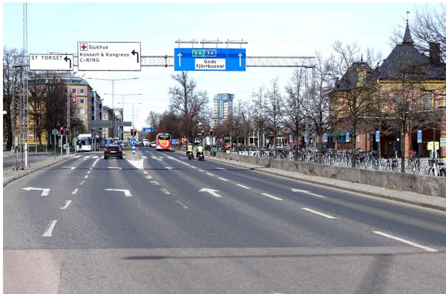
Figure 14. SMA 11 with steel slag aggregate on Industrigatan in Linköping, Sweden, 8 years old (the darker parts only). Exposed to high volumes of cars and heavy busses and laid in T-crossings. The pavement still looks good in 2025 at the age of 10 years.
