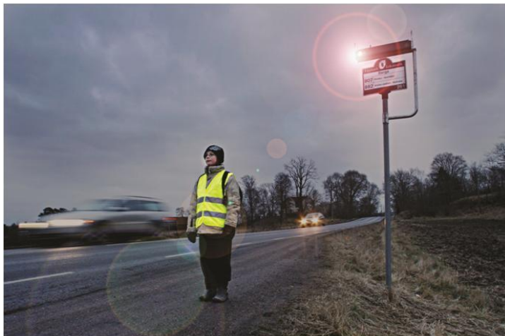
Figure 14 The IBS installed along a road in Sweden.
